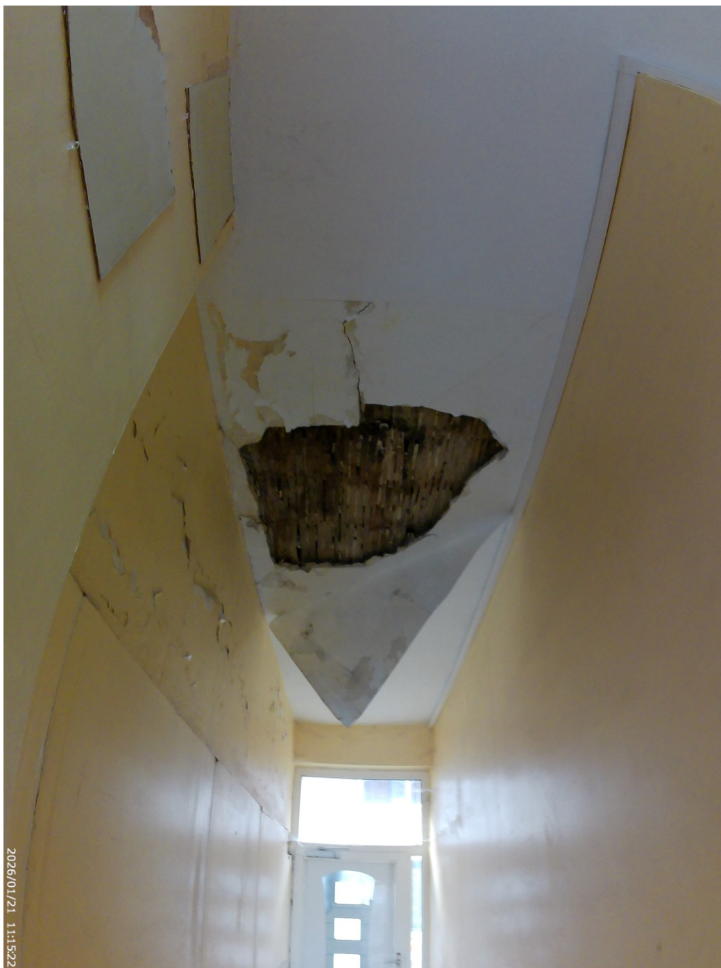
2026-01-21 - Plafond Couloir Down
